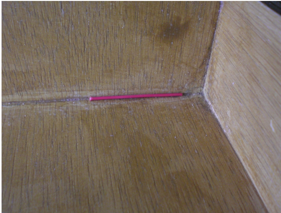
Figure 119: Wire spacer in place.
