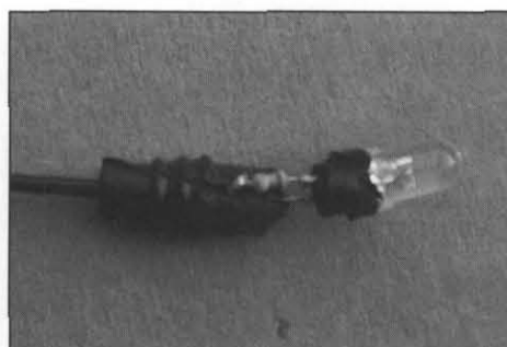
Figure 2—The LED and resistor exposed.
