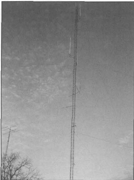
Figure 4—Inverted-Vee for 160 and 80 meters, at 150 feet!
