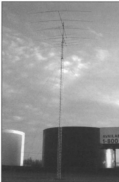
Figure 2—Tower 2, 10 and 20 meter beams.
