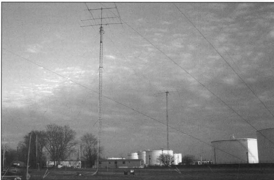
Figure 1—Mad River Radio Club antenna farm, towers 1 and 3.
