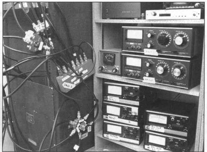
Figure 8. Patch panel and antenna switched inside the shack
