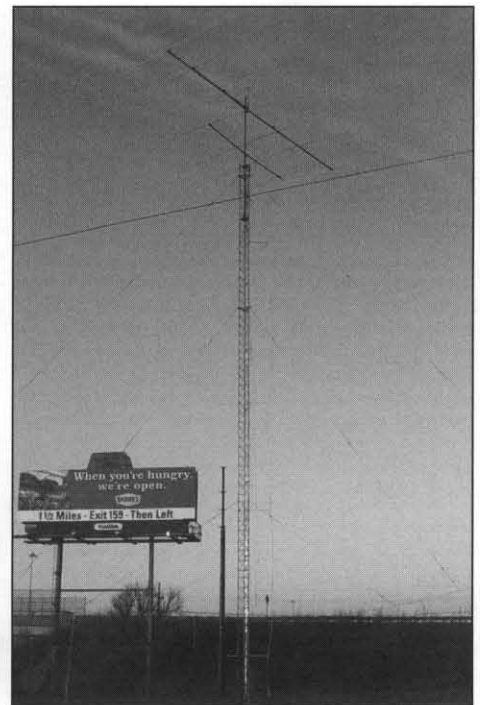
Figure 3—Tower 4, 15 and 20 meter beams.
