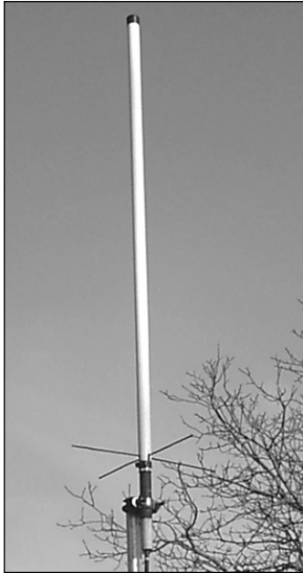
Figure 15.64: Photograph of finished antenna installed on mast
