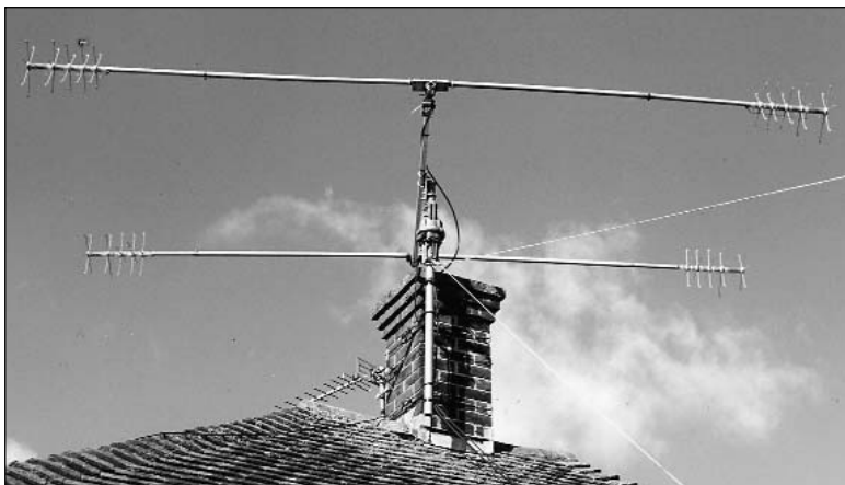
Fig 13.44: A compact two-element multiband beam
