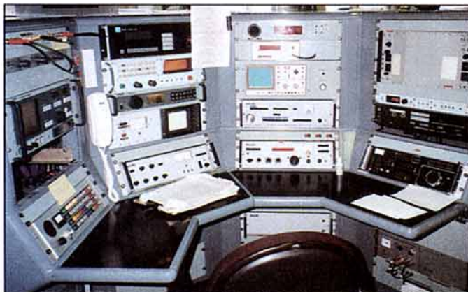
Three of these consoles allow Baldock's Terrestrial Monitoring Station to check the frequency, mode, field strength and bearing of any HF signal.
