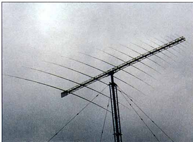
This impressive log periodic broadband antenna can be seen from the main road half-a-mile away.
