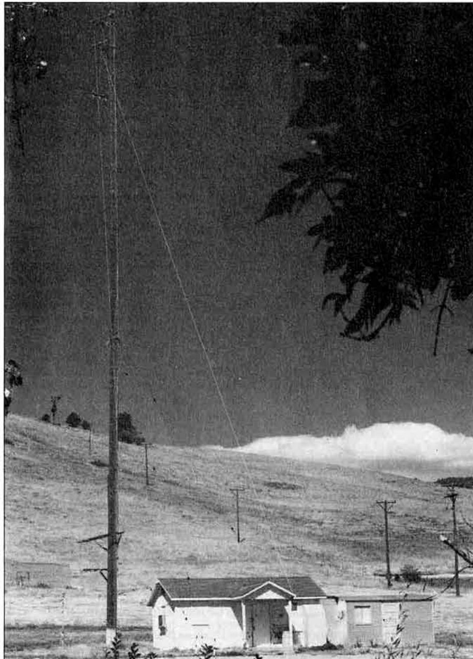
These modest buildings house the transmitting and receiving equipment of the NOAA ionosphere observatory near Boulder, Colorado. The observatory, which produces several ionograms every day, is remotely operated.
