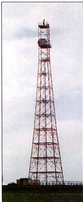
GB3TE (Clacton-on-Sea) moved site and frequency on the 2nd April and is now located on the Holland Haven Radar Tower. Locator is JO1OT and the antenna is 280 feet ASL, radiating 5W ERP. Channel = R7.
