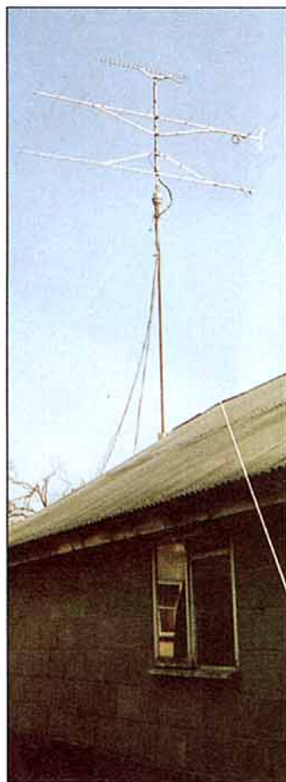
It doesn't have to be that big to work! The original G4PIQ antenna system (circa 1988) which won a useful set of contests – 14 el on 2m, 21 el on 70cm and 23 el on 23cm at 30ft.
