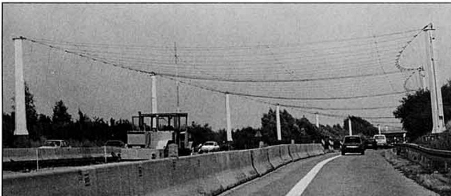
This huge Faraday screen protects car electronics from the Europawelle Saar 1.2MW MW transmitter.
