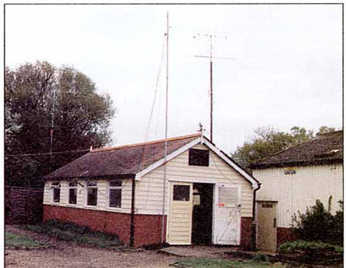
The aerials were mounted on a Romney, Hythe & Dymchurch Railway shed.
