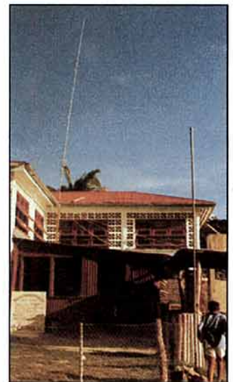
A35MR/P - HF6V roof mounted with multiband radial system in place. The shack is underneath.
