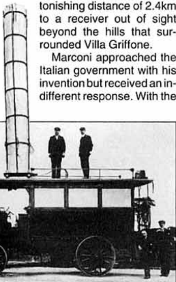
The first /M operation in 1901. Aerial is a 25ft zinc cylinder . . .
