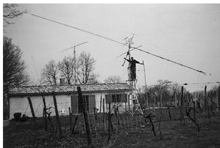
The EME 2m crossed Yagi of F/G8MBI, with its 15m boom.
