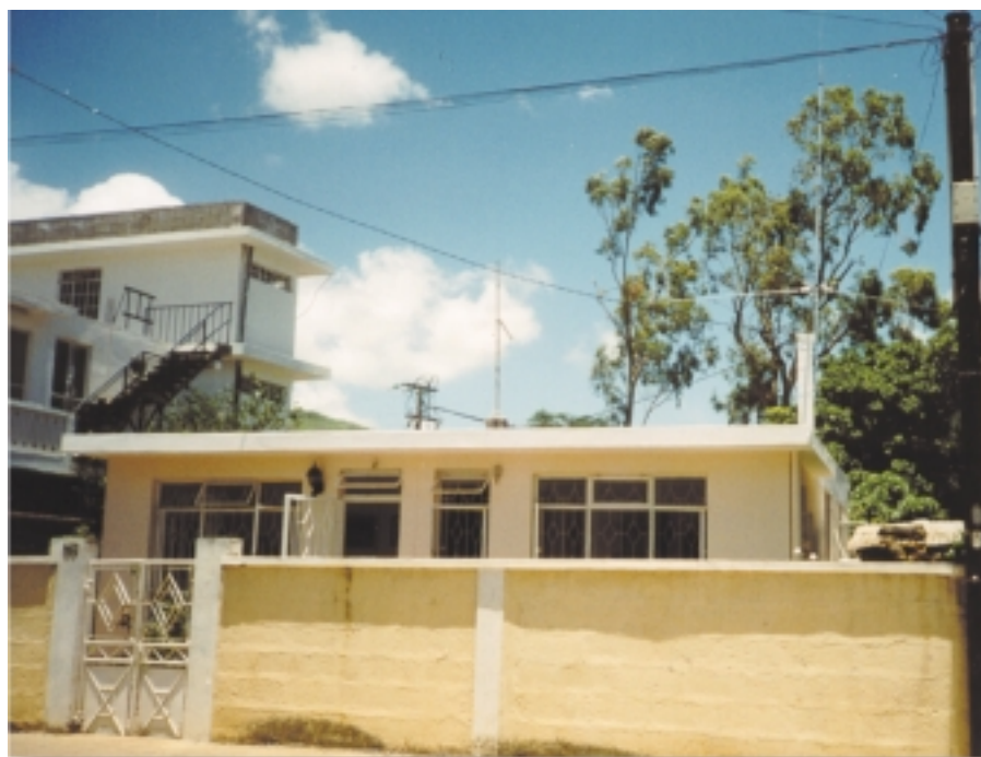
View of the bungalow and CP-5 antenna from across the street.
