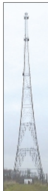
The 100m Puckeridge mast.
