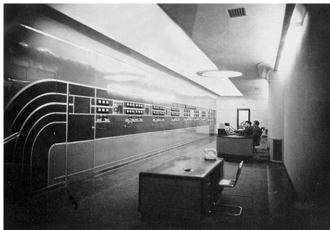
Aspidistra, which first broadcast on 8 November 1942. Built by RCA, the transmitter cost £111,801 4s 10d. It was housed in a subterranean building in an enormous hole that had been dug by Canadian servicemen. It is no coincidence that the front panel and the control room bear a remarkable similarity to old Odeon cinemas, because the same designer was responsible for both!
