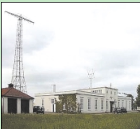
The Grimeton site of SAQ, showing one of the six 127m masts and a rather smaller cubical quad.
