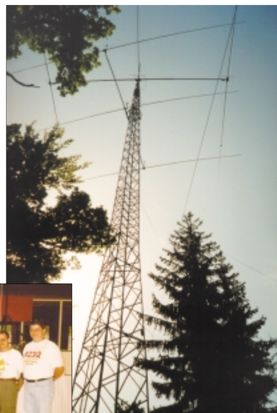
Above: 140ft tower, 80m 3-ele linear loaded Yagi at the top, 40m 3-ele full sized Yagi on ring rotator lower down. S50A.
