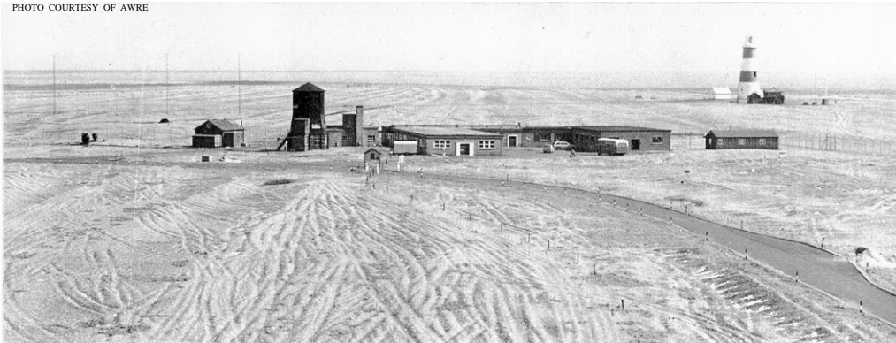
The pre-war marine radio tower which originally housed the 1920s Orford Ness beacon GFP. Also on the shingle can be seen the lighthouse which is now within the nature reserve.
