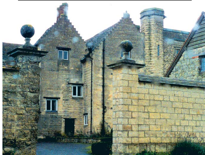
The rather forbidding aspect of Creslow Manor House.
