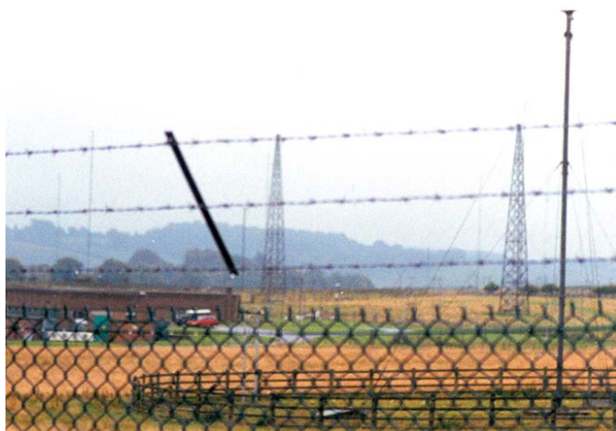
Some of the antennas at Edlesborough: a log periodic Yagi (top) and masts supporting rhombics (below).
