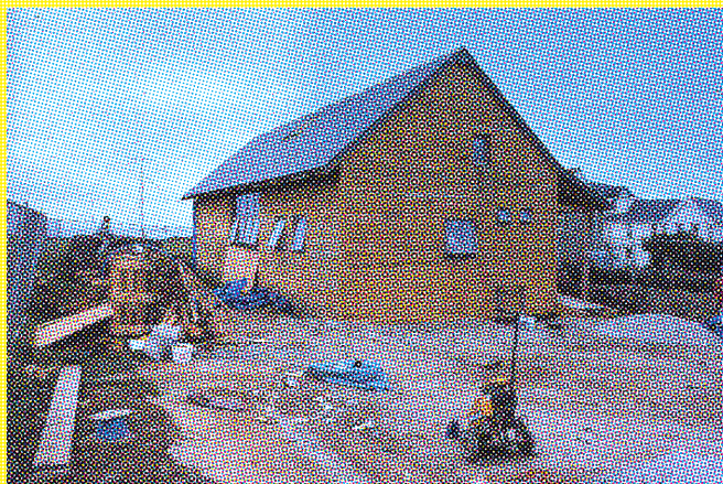
The 'Marconi Centre' building work nears completion at Poldhu.
