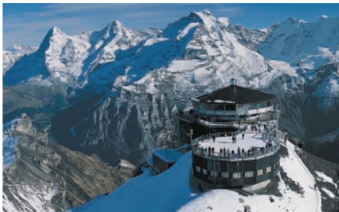
Blofeld's lair? No, the site for the HB9F repeaters.
