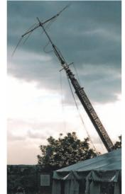
Setting up: one of the two trailer towers being erected against a stormy sky. On top, a Force 12 18 / 24MHz Yagi.
