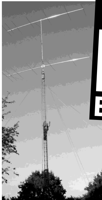
Mike G3SED's stacked pair of Trident® 6 mtr 7 element Long Boom Yagis - spaced 22ft at 75ft high
