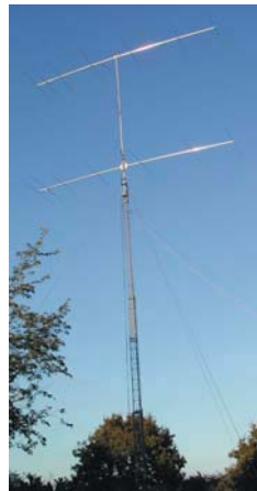
Two Trident 7-element long boom 6m Yagis spaced 22ft apart, 75ft high at the home station of Mike Devereux, G3SED.
