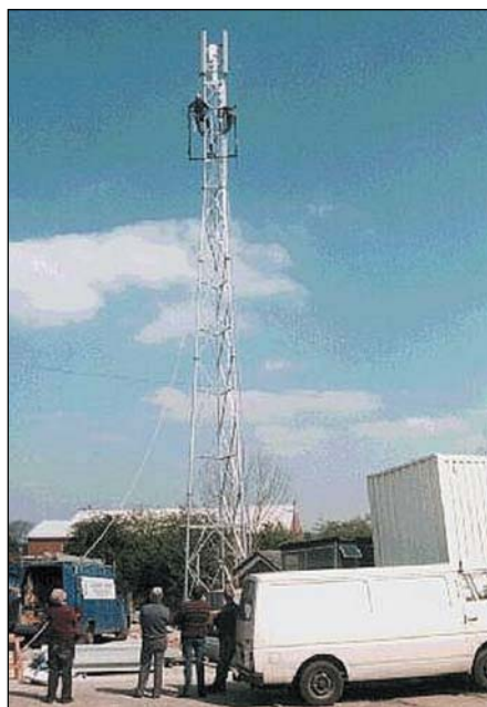
GB3HV, the Home Counties ATV Group's 24cm ATV repeater site.
