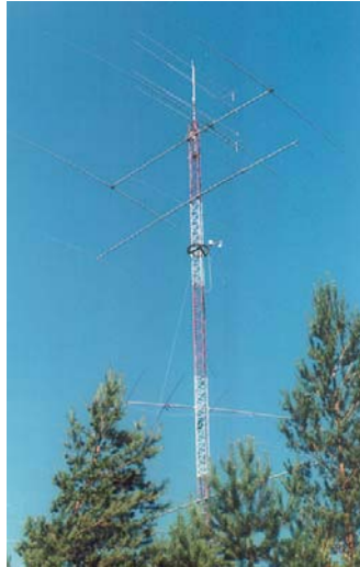
A large HF antenna array.
