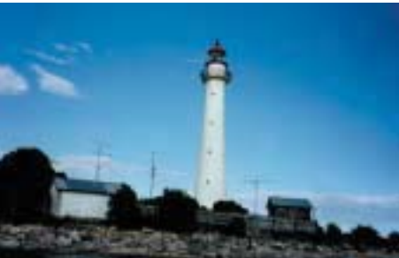
The lighthouse provides a fine mast for the low-band antennas for ES8X on Kihnu Island, Estonia (EU-178).EU-136.
