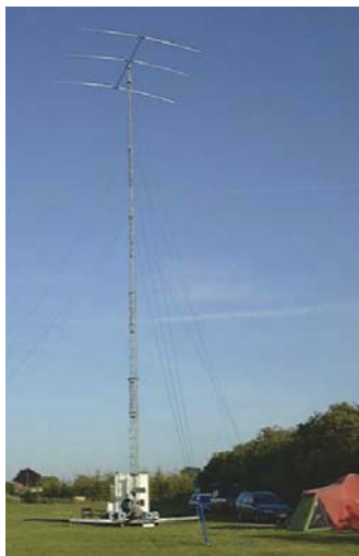
The GB5HQ 15m SSB station, located near Royston in Hertfordshire.
