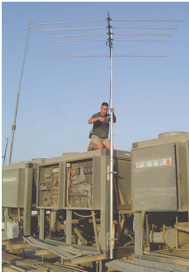
Michael Dirksen, PA5M, working on the roof of the UN building before the bombing.
