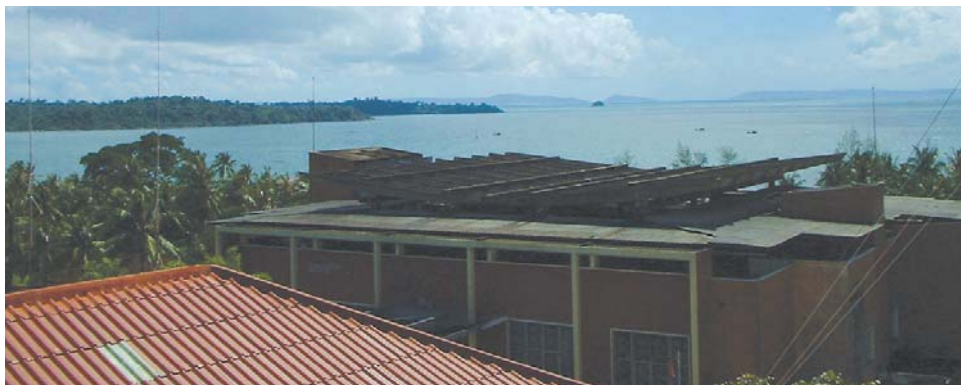
View from the roof of the XU7ACT/XU7ACU shack, looking towards the Gulf of Thailand.
