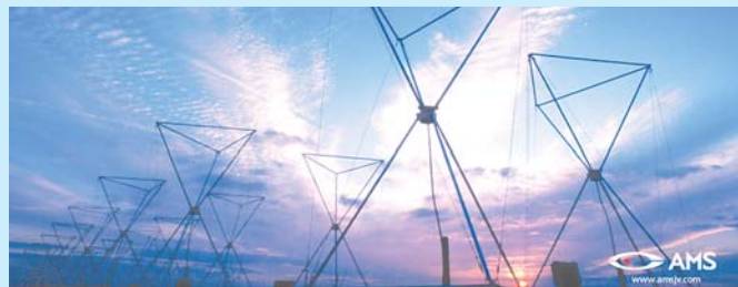
HF radar antenna array designed by Alan Boswell, G3NOQ.
