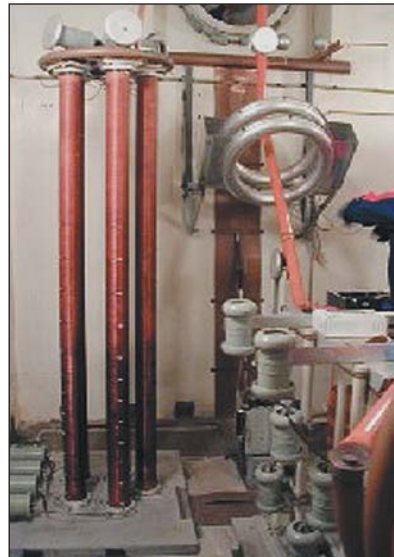
OM2TW's problems were caused by these chokes at the base of the tower (see "Big Signal" Weekend'.
