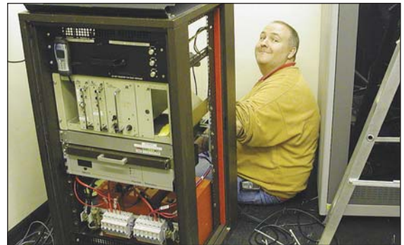
Matt, G4RKY, installing GB3FH on site.
