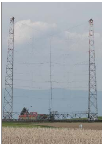
The massive former Swiss Radio International antenna system used by HE3RSI.
