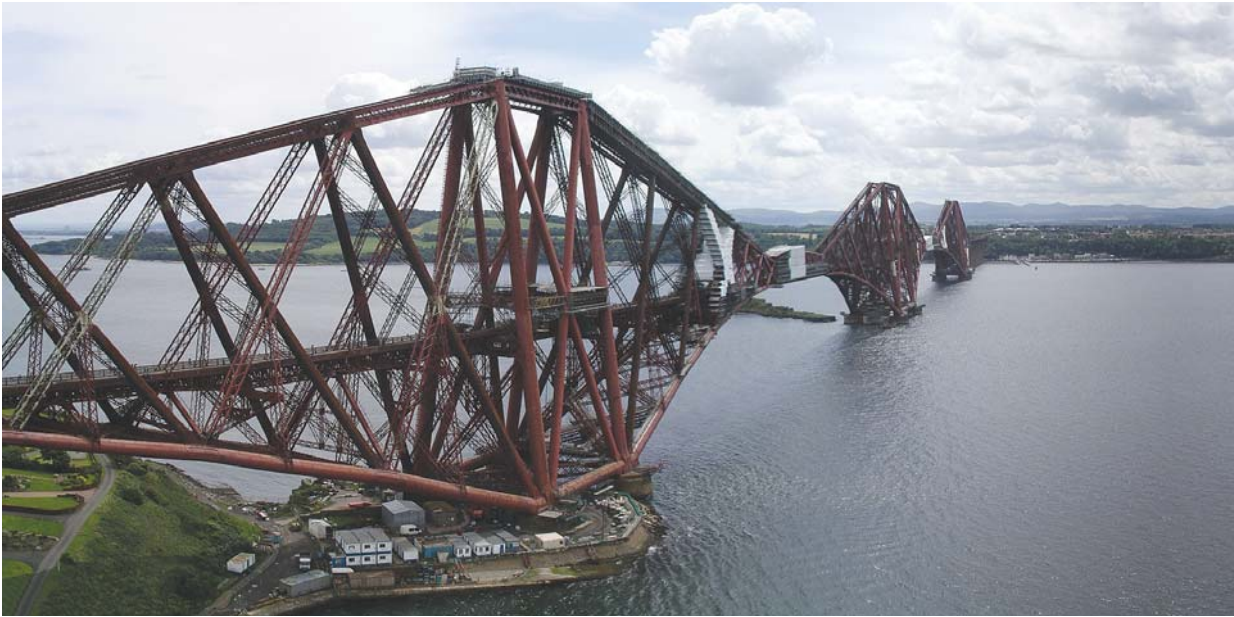
The Forth Bridge, North Queensferry.
