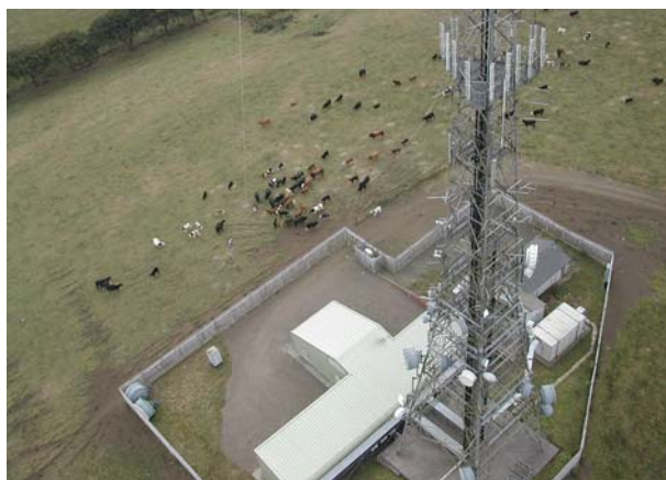
Right: Telecom mast, near Bathgate, W Lothian.
