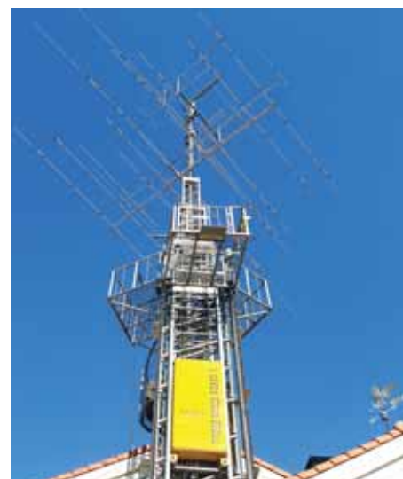
A Luso tower complete with impressive array of antennas. The one at the National Hamfest will be laid horizontal, yet it's still 12.5m in length fully retracted.
