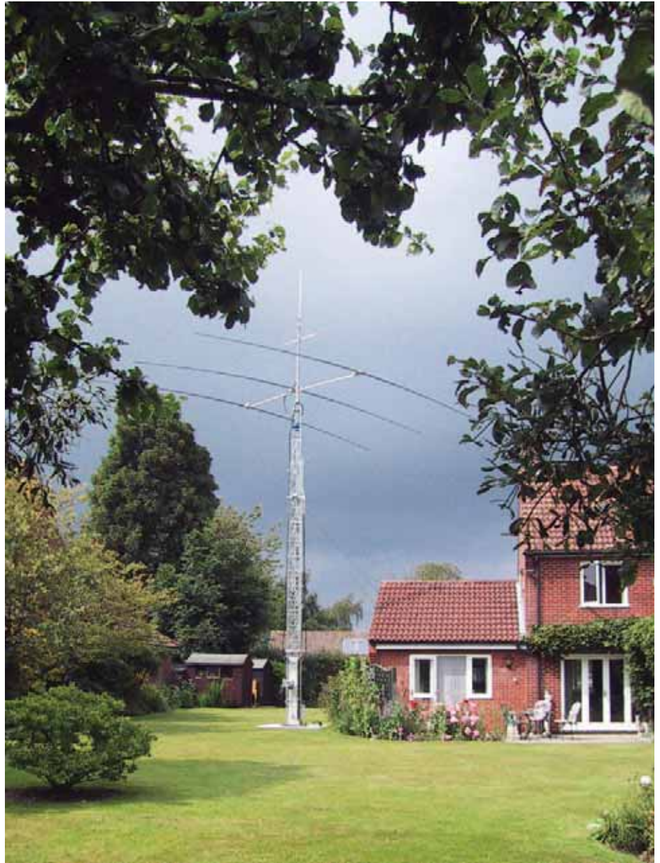
PHOTO 1: 18m mast granted planning permission on appeal. Photo courtesy G3SEM.
