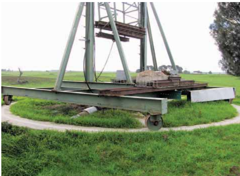
PHOTO 3: The base of VK5MC's dish showing the concrete track on which the wheels run.
