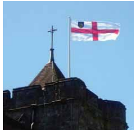
The antenna GB7MH for is cunningly disguised as a flagpole.
