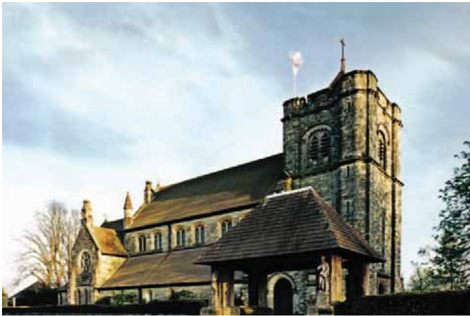
St Leonard's Church, Turners Hill, West Sussex. The flagpole atop the tower conceals the antenna for GB7MH.
