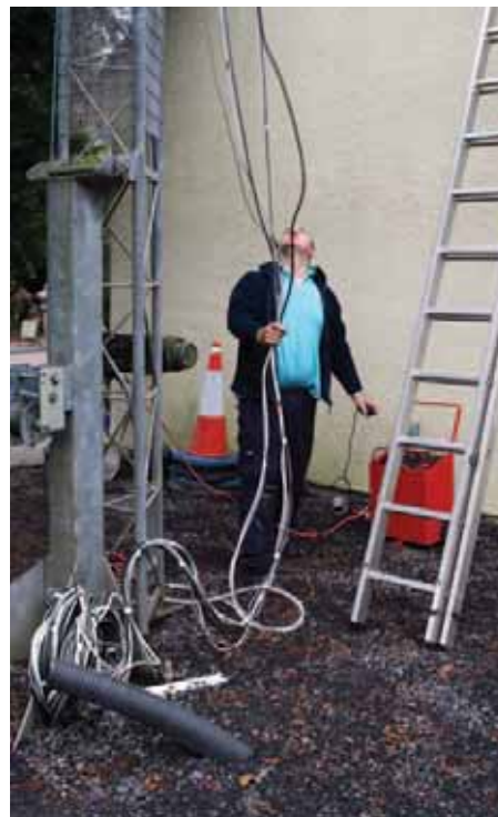
Paul, G6PZ raising the stacked 80ft tower.
