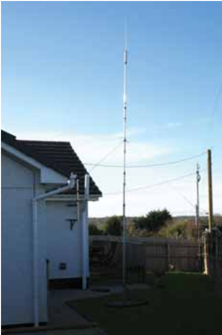
PHOTO 1: The Hustler 6BTV installation of Duncan Tribute, G1OEQ.
