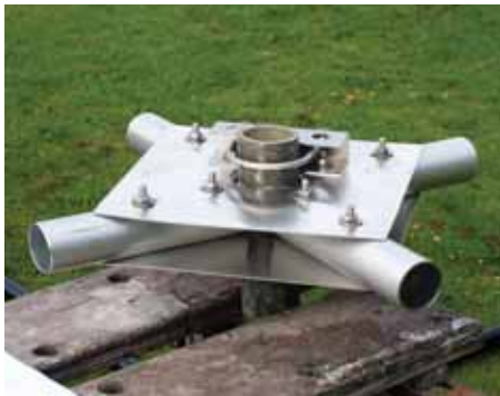
PHOTO 2: Assembling the centre joint.
