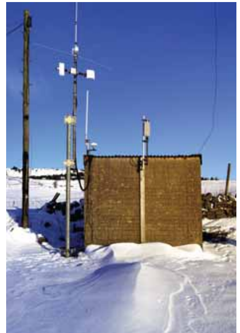
PHOTO 2: The three flat plate antennas of the 1.3GHz GB3CSB beacon, next to GB3SL, 50MHz beacon vertical antenna. Photo: GM8IHH.
