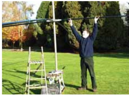
PHOTO 3: The assembled glass fibre poles were mounted on a short stub mast.
