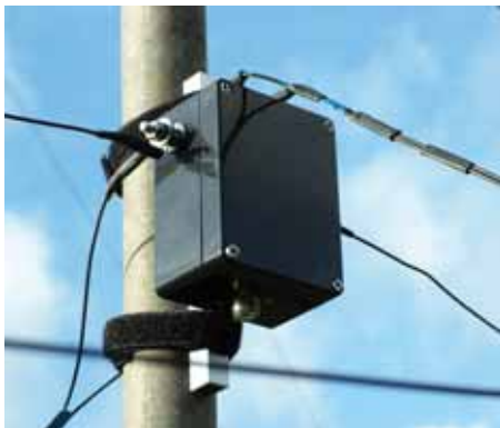
PHOTO 5: Terminating the feeders onto the balun is simple.
