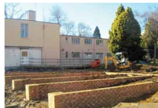
Construction continues on the National Amateur Radio Centre at Bletchley Park.
