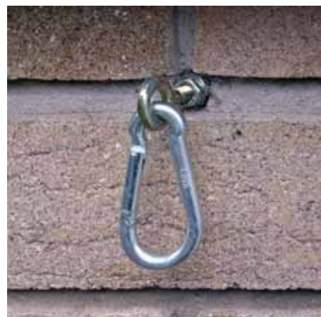
PHOTO 2: One of GW4EVX’s eyebolts. When he is going to put the mast up he clips carabiners onto the bolts, then loops the guy ropes through them.
