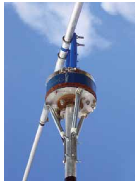
PHOTO 5: Looking up the mast, showing the foot plate and anti-rotation arms.
