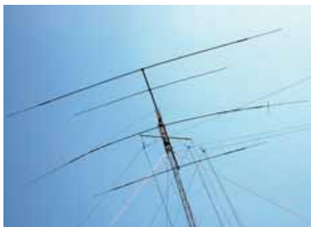
The A station antennas comprised a Strumech trailer mast with Cushcraft A4S beam with 40m extensions plus nested dipoles for 160 and 80m.
