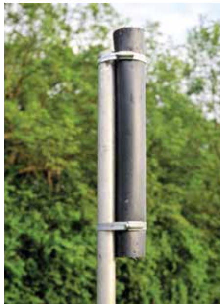
PHOTO 3: General construction of the rod support. Note how the tube protrudes an inch or so above the support pole.
