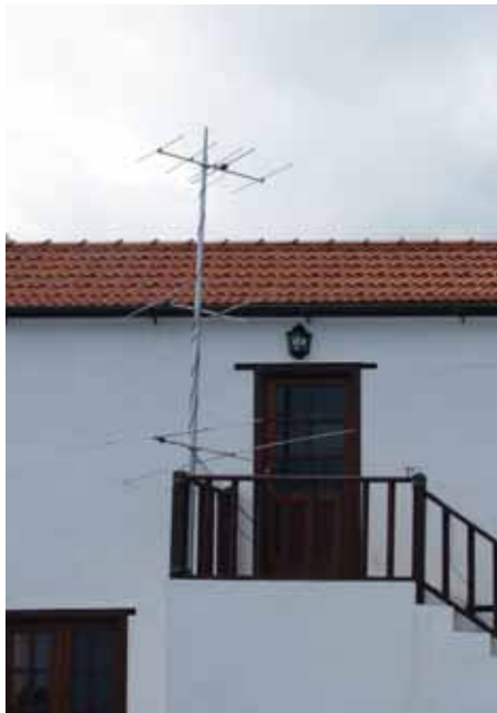
PHOTO 1: The 6m, 4m and 2m antennas at the summer QTH of EA8/DL3GCS.
