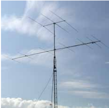
PHOTO 1: The 50MHz and 28MHz Yagis at the QTH of David Gillies, MM0AMW.
