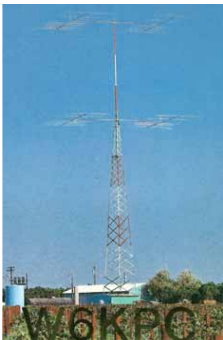
W6KPC QSL showing his 20m antenna. A third (lower) level of 2 x 6-element Yagis was added later (this card was for a 20m QSO with G3XTT in 1979).
