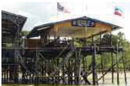
The SMK Wallace Bay school jetty was the location for our operation. The Butternut HF6V vertical was mounted on the post by the Sabah state flag to the right of the photo.
