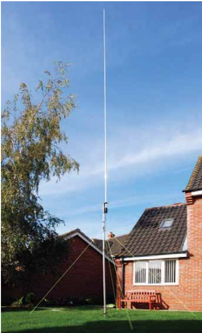
PHOTO 1: The Moonraker GP2500 mounted on a 10ft pole, suitably guyed.
