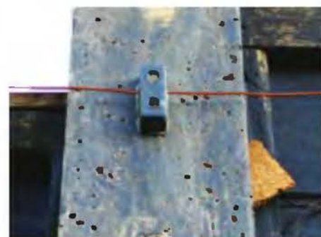
PHOTO 1: A furniture block, glued to the fence post, makes a decent insulator.
