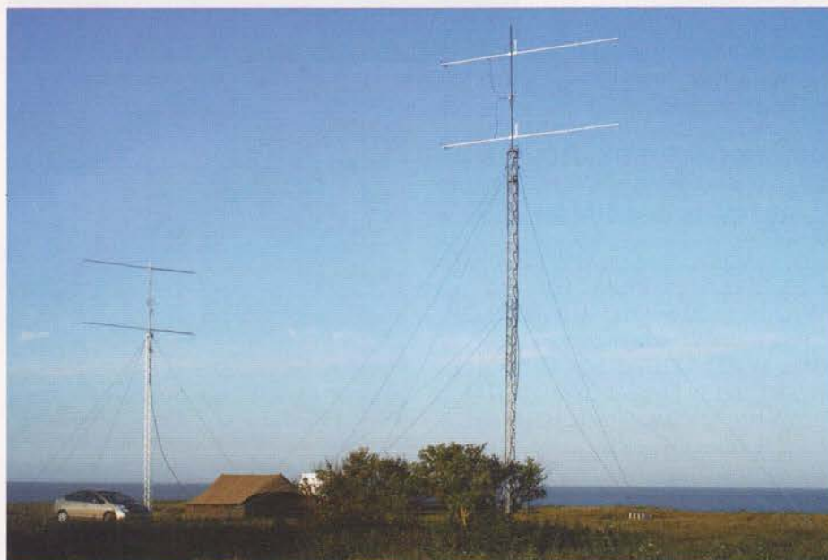
PHOTO 1: The 144MHz antenna systems used by the Colchester VHF Contest Group, G0VHF.
