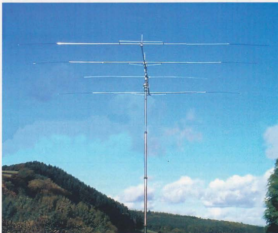
PHOTO 15: My completed PICaYAGI in service on 15m.
