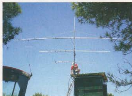
SV8CS finalising the installation of his 50MHz 7-ele WOS LFA Yagi at his green station.
