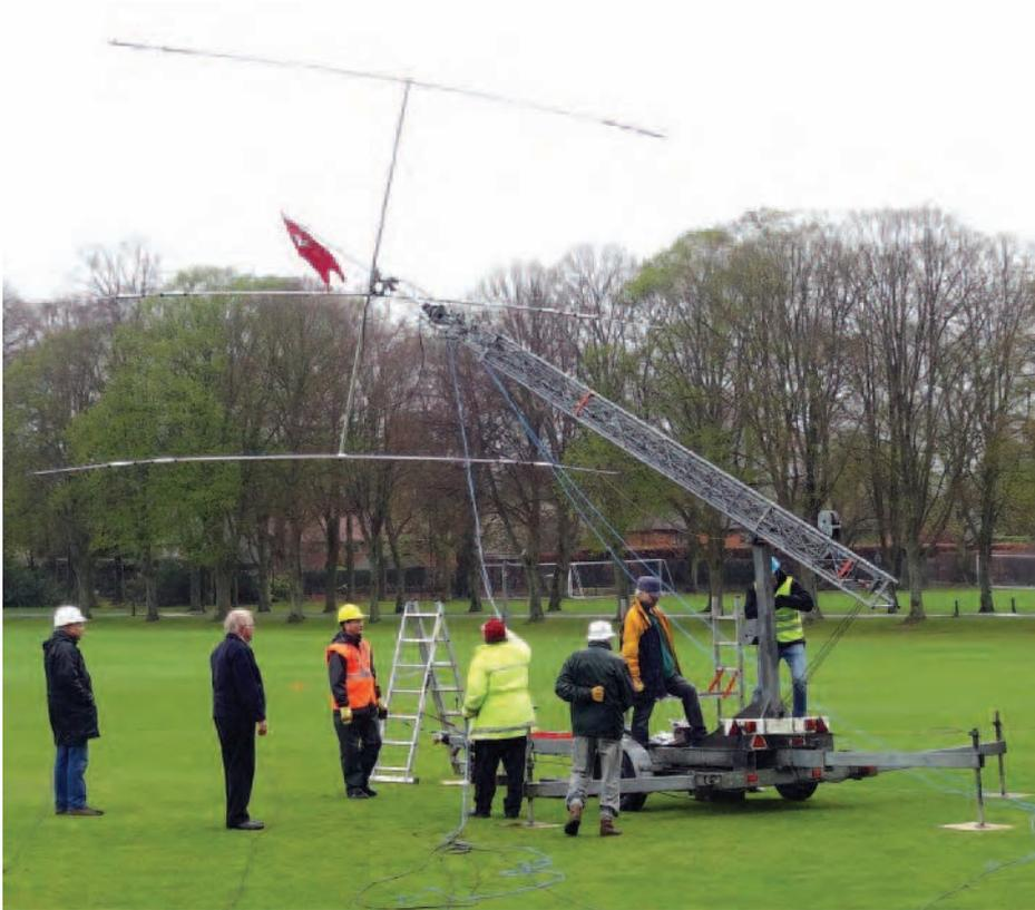
One of two 60ft trailer towers supporting dipoles for 80m and 40m, a trap dipole for the WARC bands 30m-17m-12m, a 3-element Yagi for 20m and a 3-element tribander for 15m-10m.
