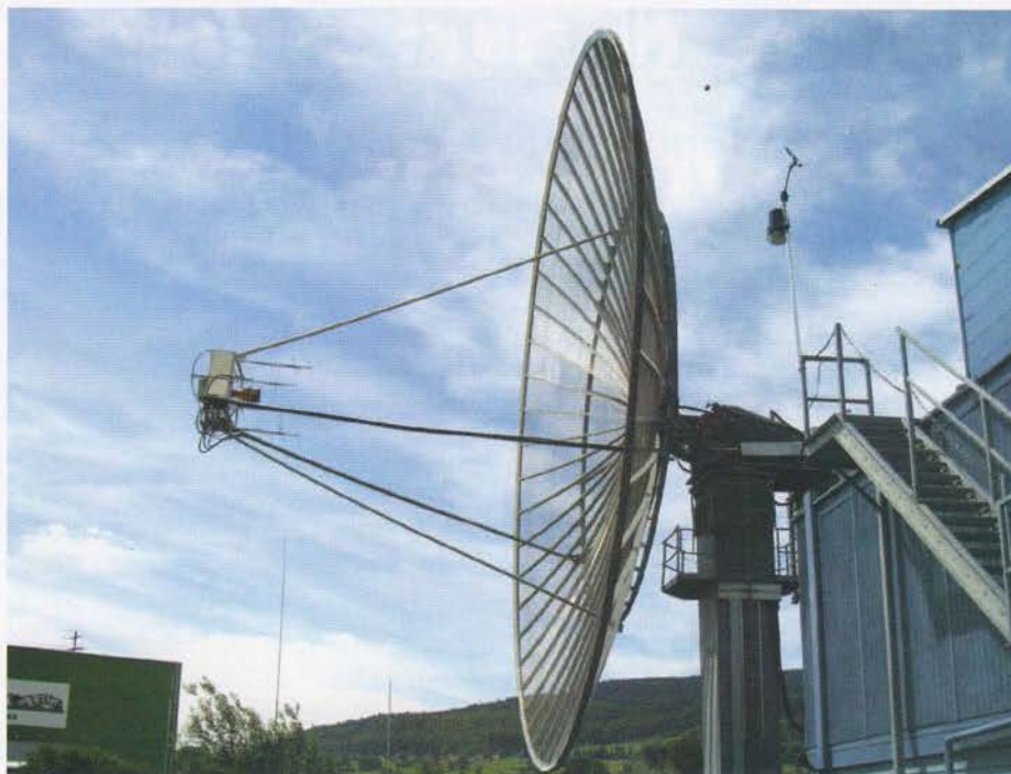
PHOTO 3: View of the HB9Q 15.1m dish and radio room.
