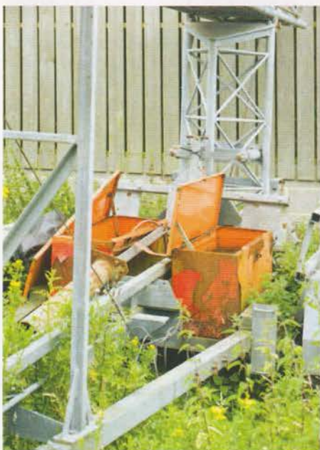
The equipment boxes are either sand blasted and re-sprayed or replaced completely.
