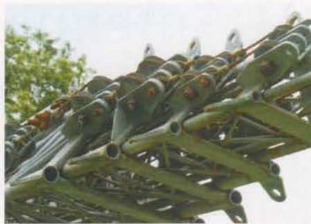
A tower awaiting refurbishment.
